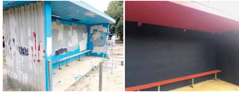
Guinther Park Dugout - Before and After Clean-Up
