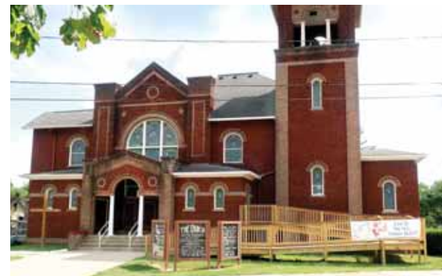
The New Handicap Ramp at TCoTB
