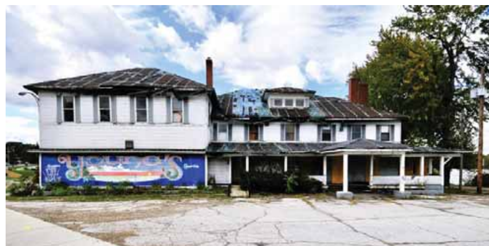
Young's Restaurant in 2010 Prior to Demolition
