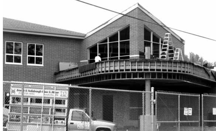
The New Sam Salem Community Learning Center (still under construction).
