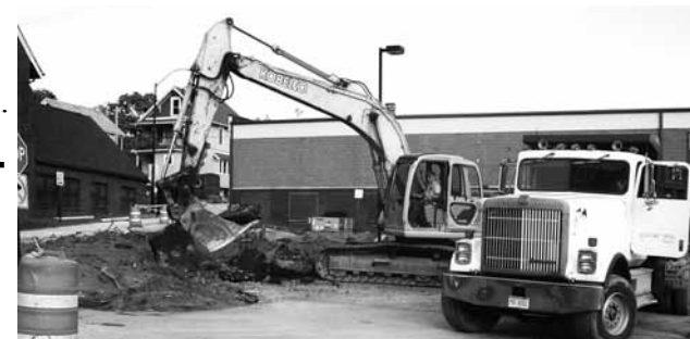
Construction starts on the new library
