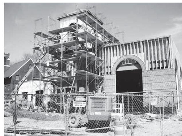
The Tower is near completion
