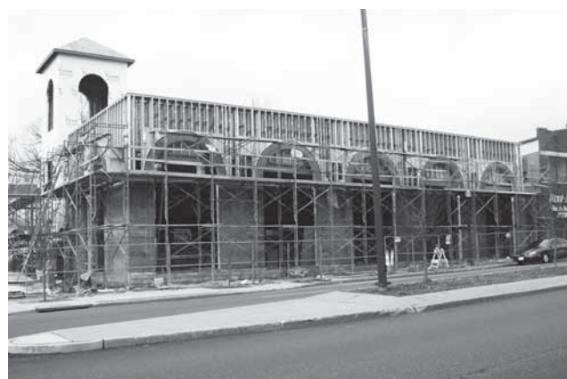
Laying bricks for the new Kenmore Library
