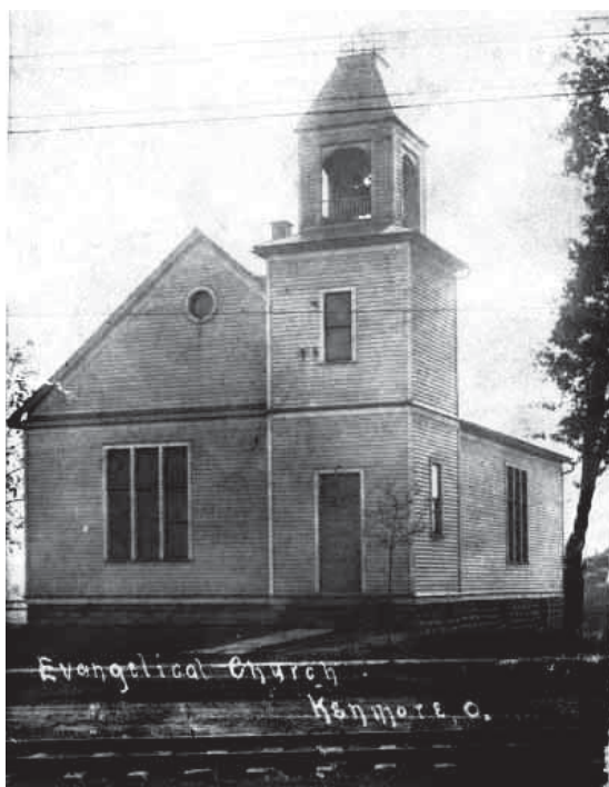
Wooden church that preceded the current Church on the Boulevard
