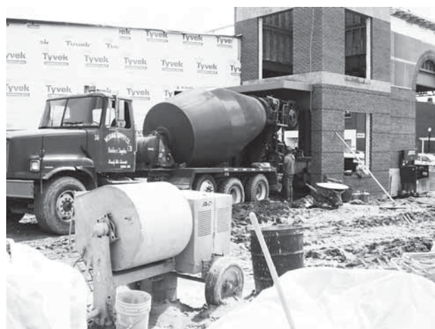
Trucks come in to pour the cement foundation
