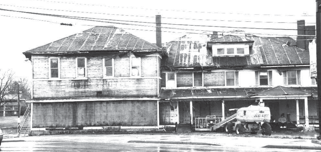
When the siding was removed, the words "Young's Hotel" were revealed below the windows on the front of the building.
