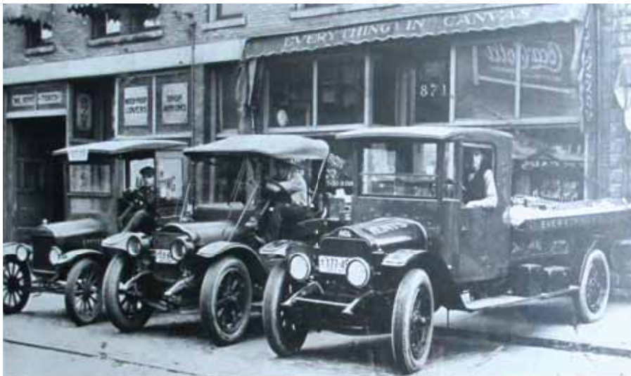
First Location of South Akron Awning on South Street
