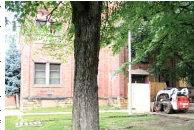
Heminger Ready for Demolition
